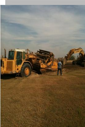
Levee improvements recently completed at the Turnipseed Basin Banking Project site included reconstruction of selected banks to increased capacity.
