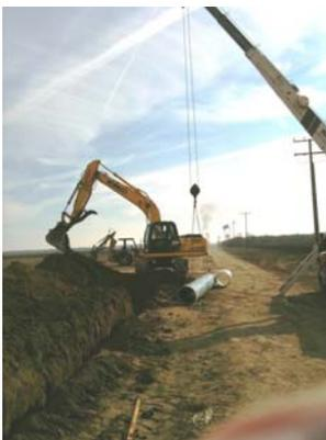
*District staff installing new pipeline that will tie in new recovery well water to the DEID distribution system.*
