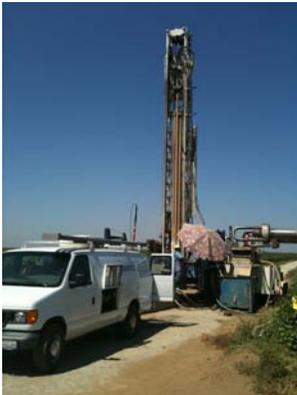
*Groundwater monitoring well being installed near the Turnipseed Basin project. A total of five dedicated wells were installed this fall.*
