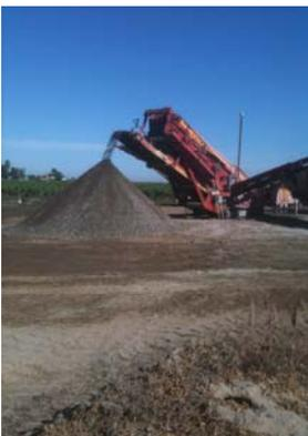
*The collection of old concrete pipe and debris was piled, grinded and reduced to road base this summer. The base rock will be used on the main interior road in the basin to allow year-around access.*
