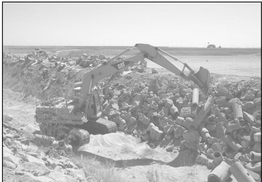
**An excavator being used to install concrete debris from previously renovated turnouts on selected banks of White River. The slopes were previously unprotected and subject to potential erosion.**
